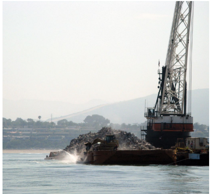
Figure 5.10 Building an artificial reef. Photo supplied by the authors.
